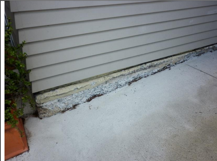
Weatherboards on a cavity with exposed footing shown below.
